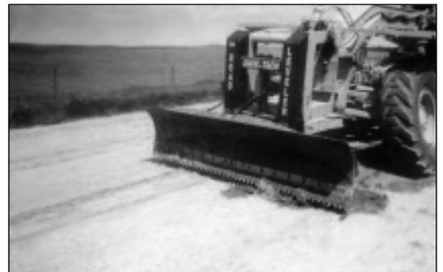
can be used effectively on a front-mounted dozer blade. The operator can drop the dozer to cut out washboards and use the moldboard to shape the area.
